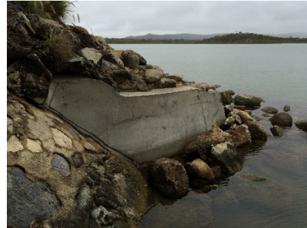
Repaired Batter Wall
