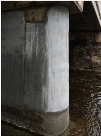
Pier Nosing Repairs
