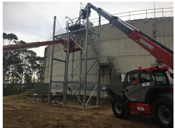
New staircase installation
