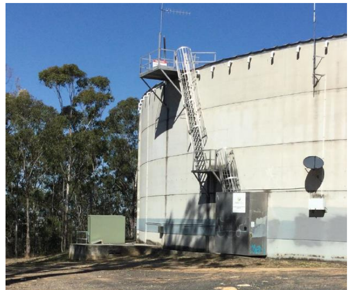
Existing staircase before removal
