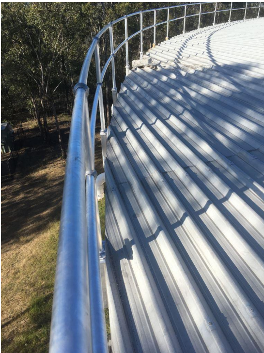
Railing along roof edge
