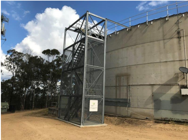
New staircase after installation
