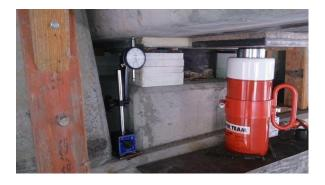
Each girder was then evenly lifted at a continuous rate to a point where each bearing can be easily accessed and grouted. These were then grouted with Chemrite Epoxy Pad grout. Small gaps were grouted with a low viscosity crack injection epoxy.
