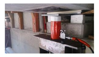
A 20mm support plate was placed on top of the jack to evenly distribute the load and these were grouted with fast curing Chemrite CR-FC grout.
