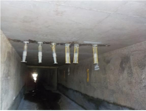
Structural crack injection
