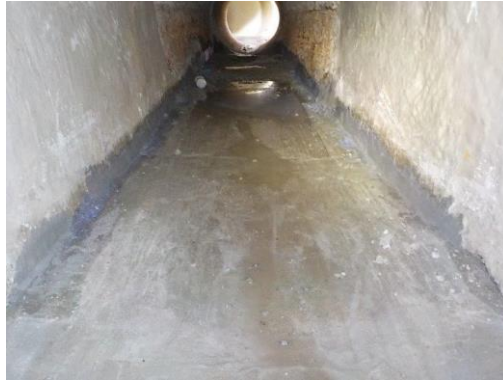
Floor screeding to provide improved flow and easier access
