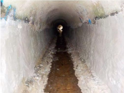
Badly eroded culvert walls reinstated with epoxy render material
