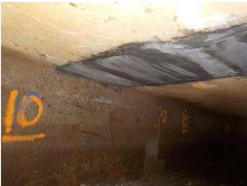
Repairs to soffit
