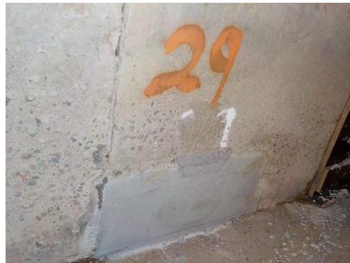
Reinforcement repairs to the walls
