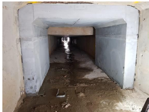
Strengthened culvert section as per design provided
