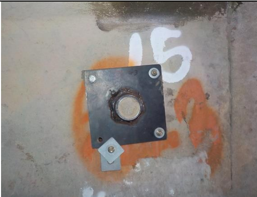
Filling voids behind the culvert walls
