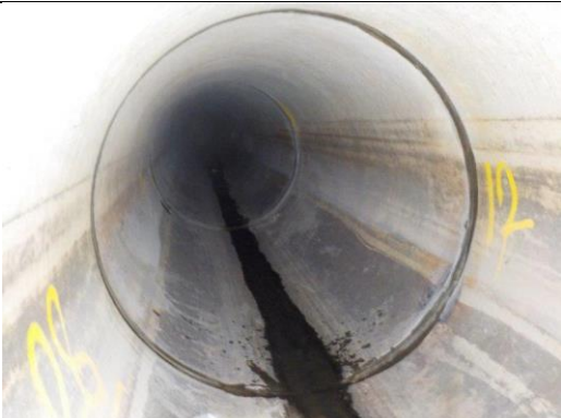
Joint remediation works
