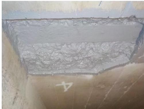
Epoxy coating in low steel reinforcement areas.
