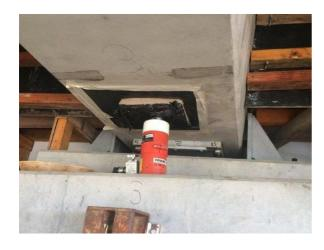
A 20mm support plate was placed on top of the jack to evenly distribute the load and these were grouted with fast curing Chemrite CR-FC grout.
