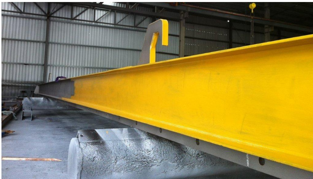
Photo of a beam being coated with Dynaciv protective epoxy coat
