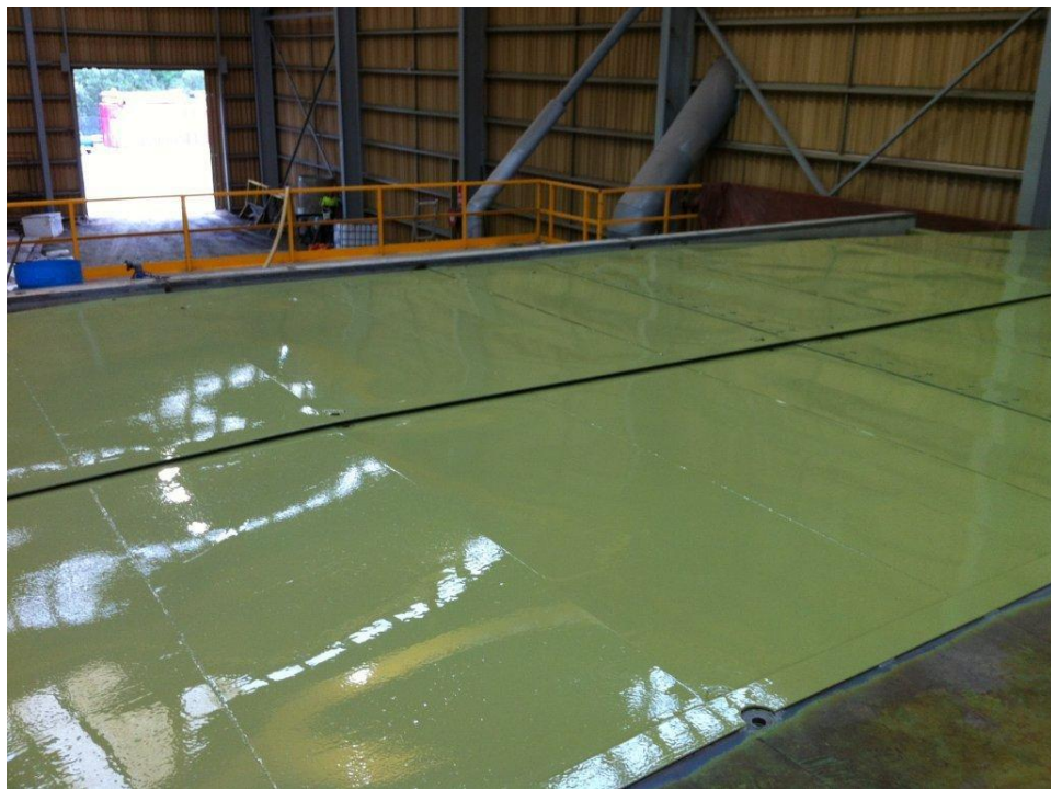
Photo showing half a door already coated
