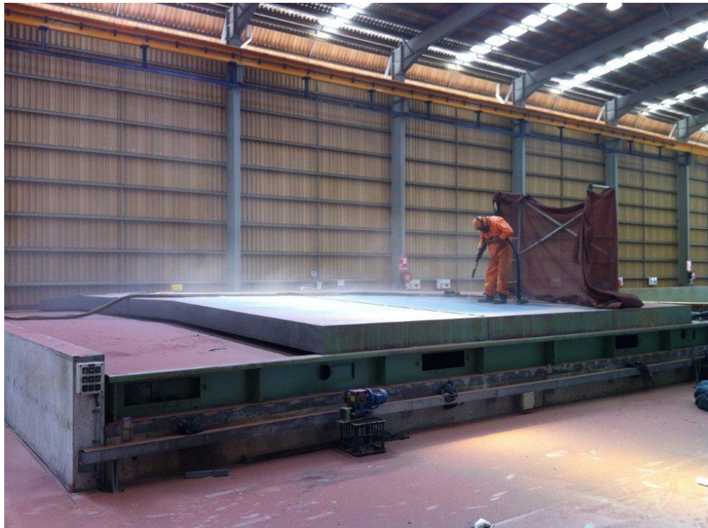
Photo showing abrasive blasting of the oven doors
