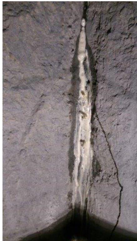
Work was also done on the surface in both portals, vent towers and other associated structures such as bridges. The photos below show concrete repairs done in the entrance to the western portal.
