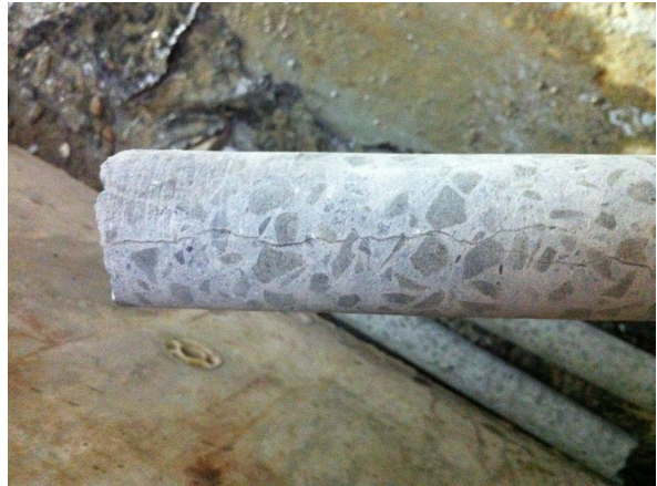
As most of the work was done underground, groundwater was a common problem that had to be managed. Epoxy Solutions adopted various methods to inject a closed and open cell foam in various places. This was often done to slow or stop water, so a more permanent solution could be implemented.
