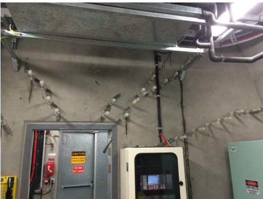
The photo below shows a deep beam below the ICB that was successfully injected using various methods, including high pressure.
