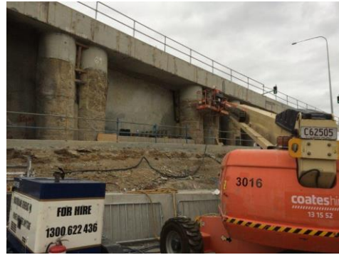
Below: The Russell Terrace bridge that we lifted/jacked to install the bearing grout.
