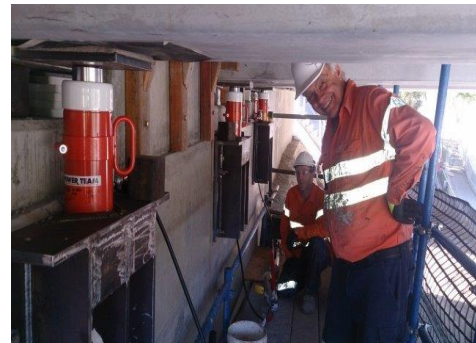
Below: The Russell Terrace bridge that we lifted/jacked to install the bearing grout.
