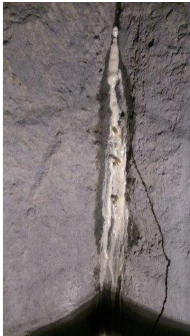
Above: Foam slowing water flow into the work site
