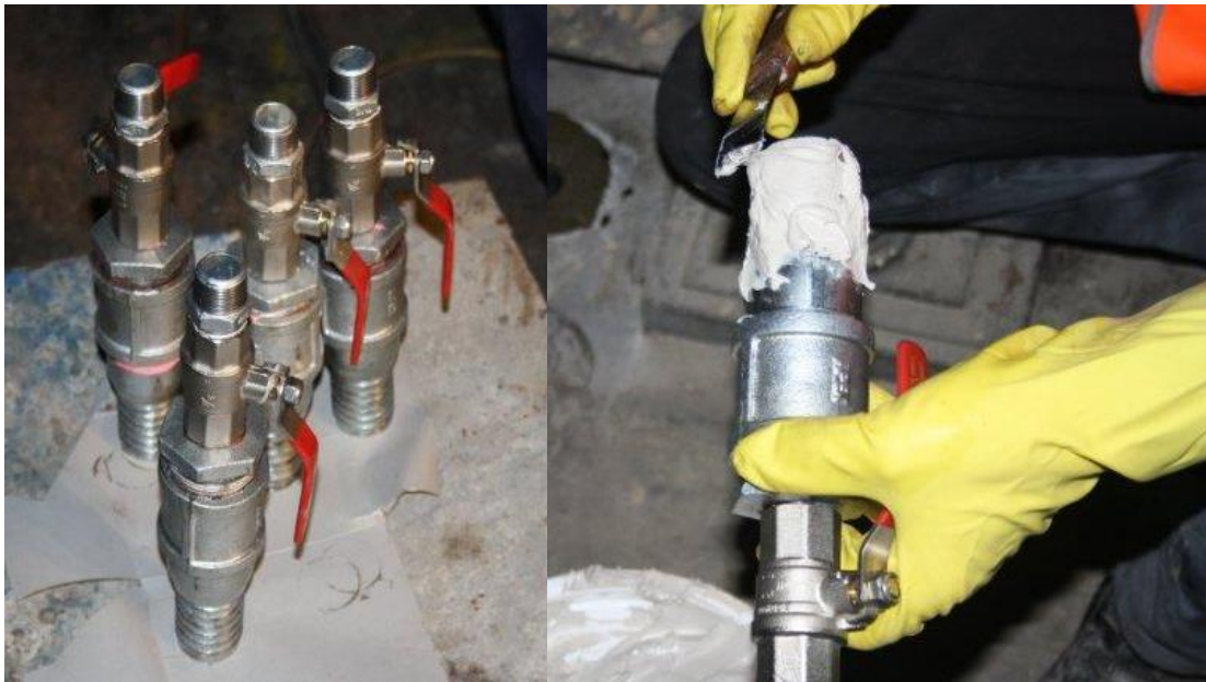
Showing the grouting of the coupling with CHEMRITE® Epoxy Paste
