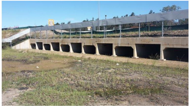
Culvert C2010 (Southbound)
