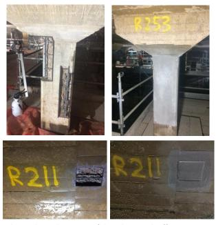
Photos above show some of the column and soffit repairs.
