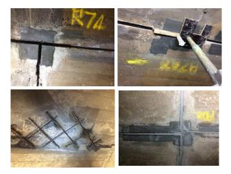
Photos above show repairs along the new expansion joints, corroded reinforcement bars replaced, voids in new expansion joints injected with a polyurethane and joints filled with joint sealant.
