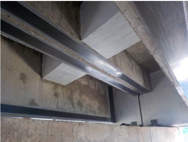
Below: Completed bridge end diaphragms
