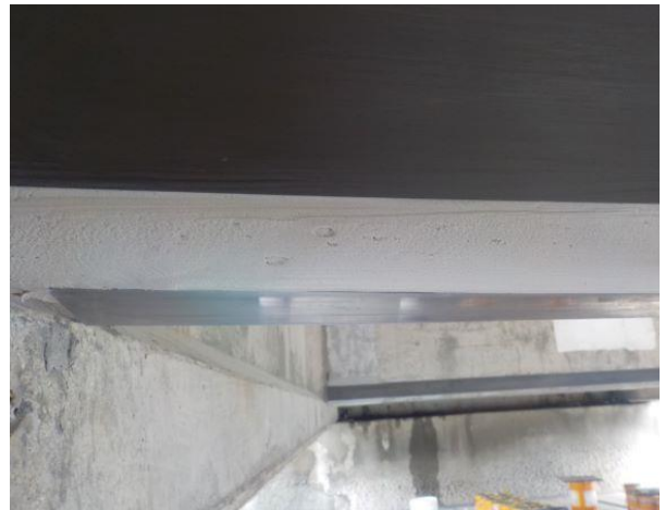
Below: Corners rounded in preparation for CFRP wrap
