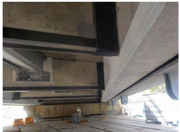
Below: CRFP laminate and wrap applied to bridge diaphragms
