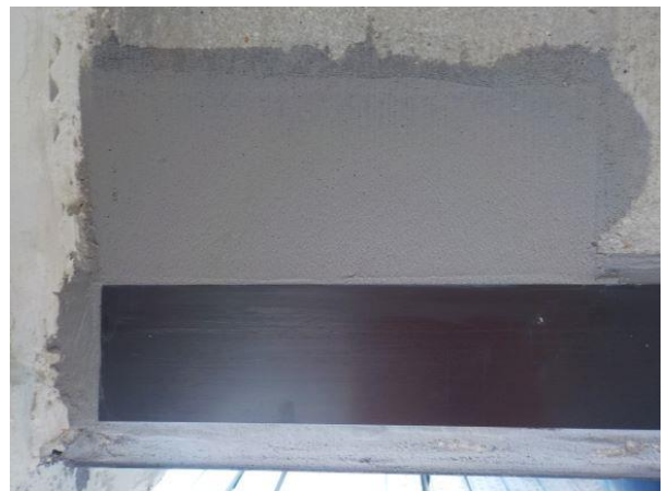
Below: Concrete profiled to meet strict CFRP specifications
