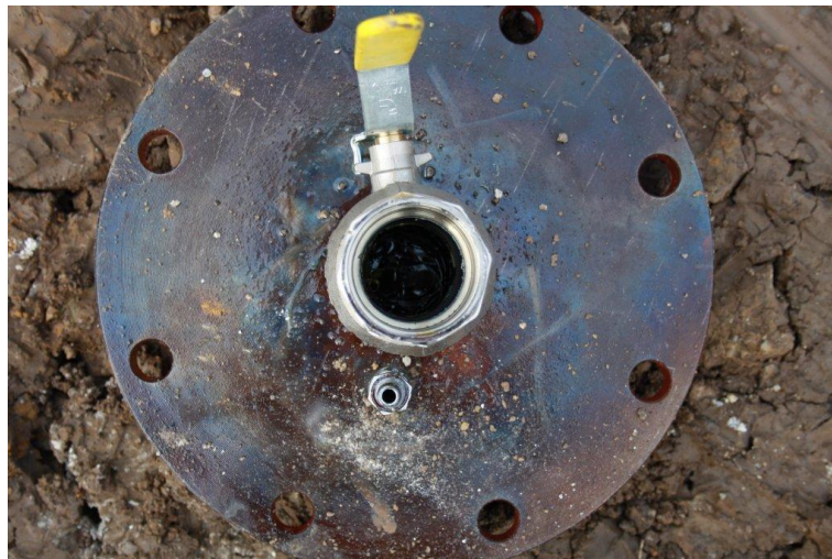
Collar cap, open valve and surface of the epoxy
