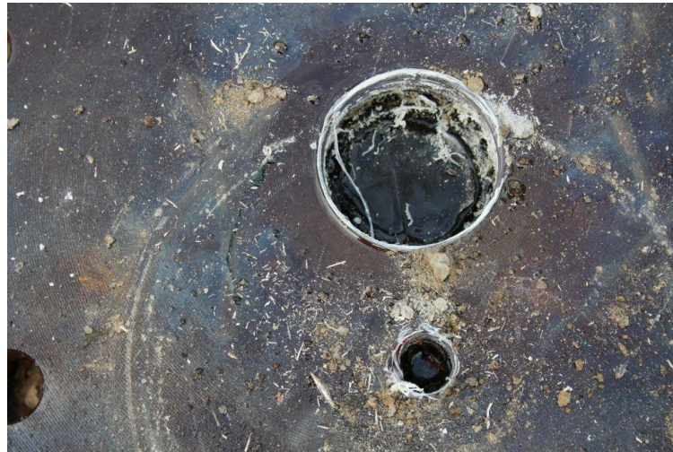
Close-up of the collar cap with the valve and air inlet removed
