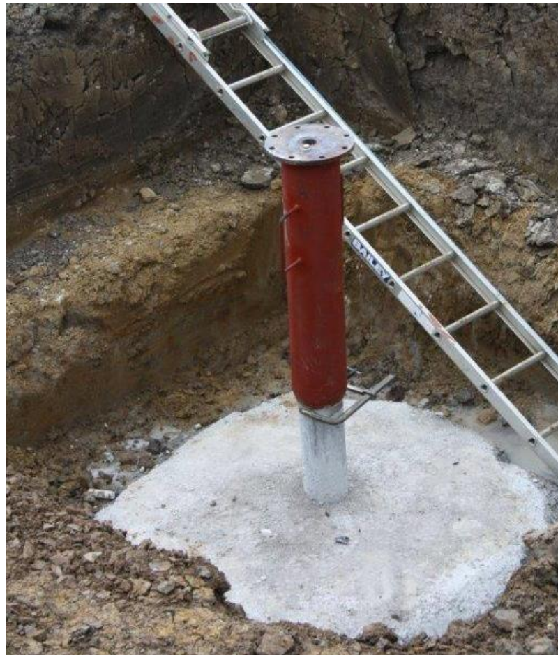
Well collar before welding
