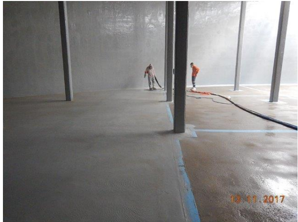
Photos: Polyurea membrane application and testing
