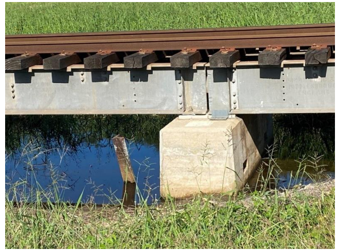
Typical work site and existing bearing
